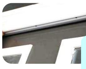
If the gap is uneven, use a **weather strip**. It has a rubber seal (like on your fridge)
