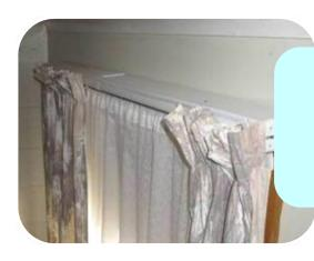
A **ledge pelmet** sits on top of the curtain rail, out of sight. It can be made from thick cardboard, foam, or wood – anything that blocks the space
