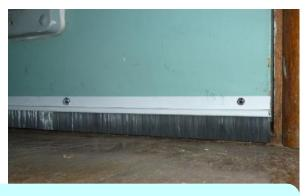
For the bottom of outside doors, you can use a **weather seal or brush strip**.
