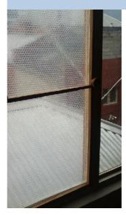
Window **insulation film** can help keep warm air in. "Clear Comfort" is a seethrough plastic which you attach to your window frame and then shrink it to fit with a hair dryer. Or try using bubble wrap for instant double glazing! Just hold it in place with velcro tabs or a light mist of water.
