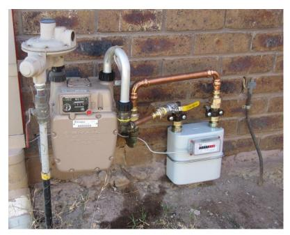
Figure 7: The existing gas distributor's gas meter (left) plus an additional gas meter (on right) which was installed to monitor gas use onsite
