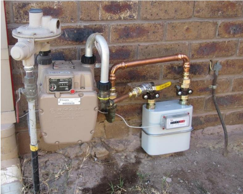
Figure 7: The existing gas distributor's gas meter (left) plus an additional gas meter (on right) which was installed to monitor gas use onsite
