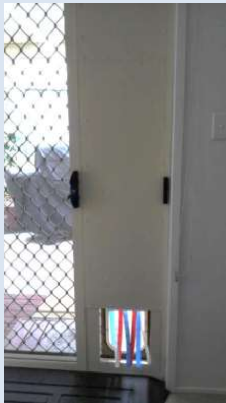
Figure 4.59 Glass sliding door with wooden panel placed in track, blocking airflow except through cat flap.
