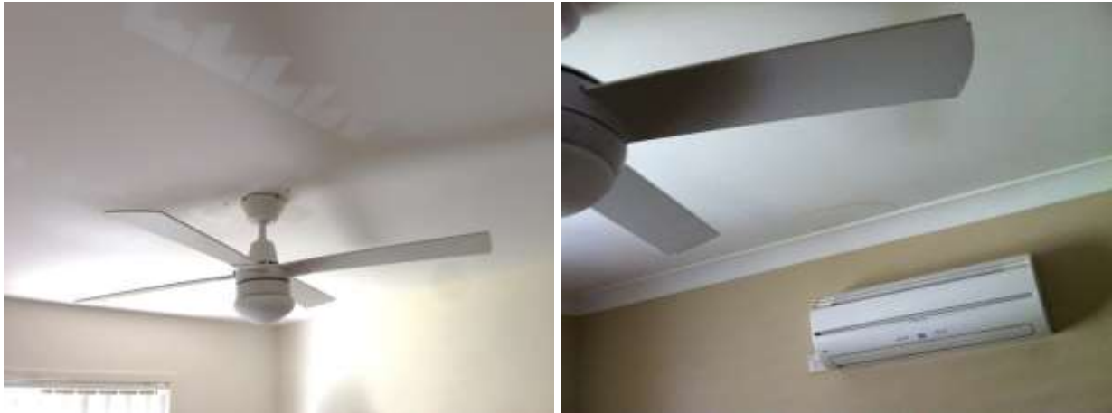
Figure 4.58 Typical ceiling fan and reverse cycle air conditioning retrofits.
