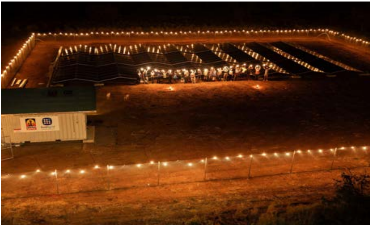
Image: Marlinja microgrid launched and lit up at night, July 2024.
