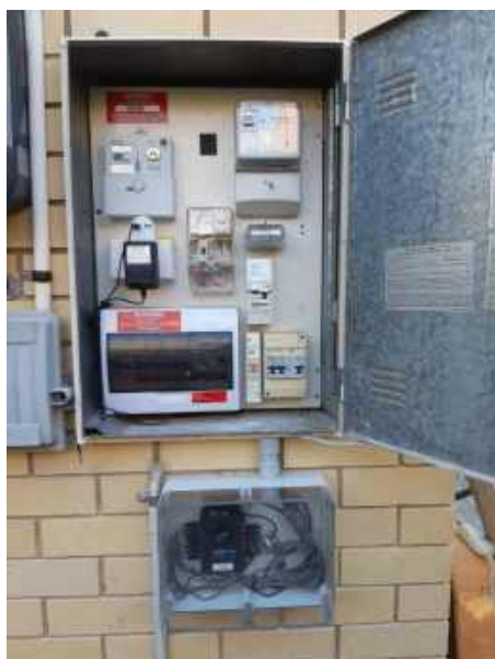
Figure 2: Phisaver installed in Perspex enclosure below meterbox. CT's are clamped behind the meterbox to circuits and main incomers.
